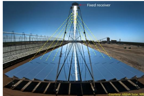
Linear fresnel reflector (LFR)
